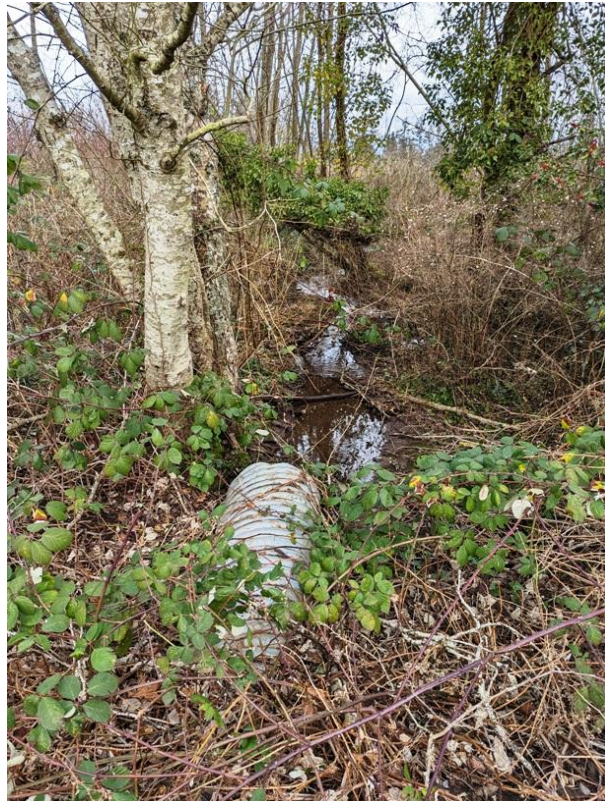
Photograph 6. January 23, 2025. View of culvert discharging ditch flows from Superior Road onto the subject property.
