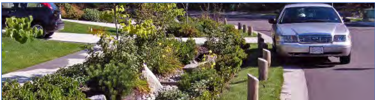
Figure 21: Storm water source controls – infiltration swale.
