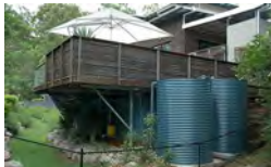
Rainwater capture tanks on a single-family home
