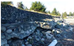
Erosion along seawalls
