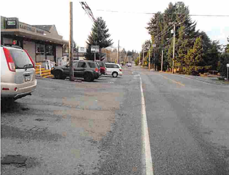
Example of 'wide' shoulder where shoulder blends with parking
