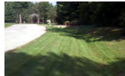
Grass stormwater swale along roadway
