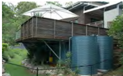
Rainwater capture tanks on a single-family home
